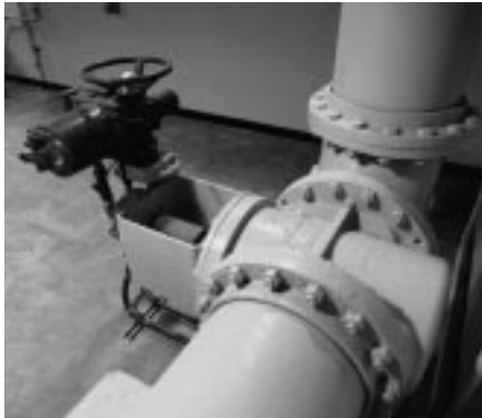
18" Cam-Centric® plug valve with motor actuator.
