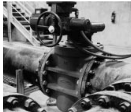
18" motor actuated Cam-Centric® plug valve.
