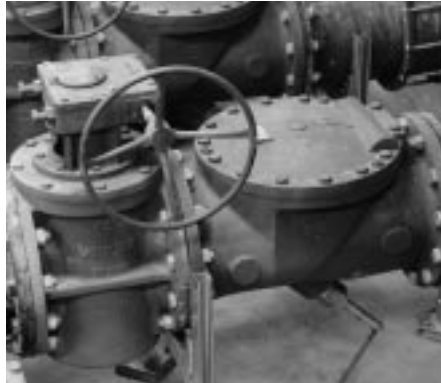
14" Cam-Centric® plug valve with Val-Matic® Swing-Flex® Check Valve.
